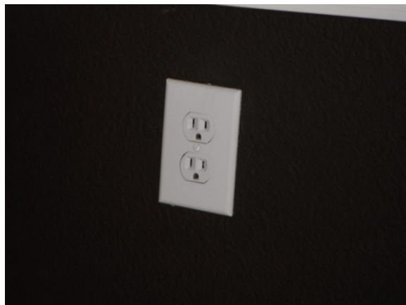
Electrical outlet is loose in Media Room
